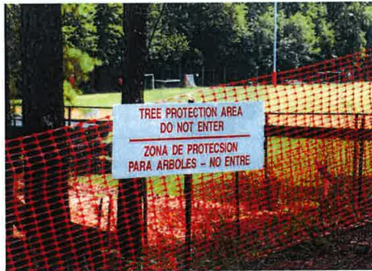
Figure 1. Tree protection zone. A protected zone preserves roots and soil and keeps branches clear of contact with construction equipment and materials.
